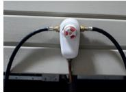
Screw on the gas pipe couplings. Fit the cover.
