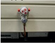
Fit the pressure reducing valve/inverter using the two screws.
