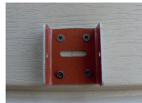
*Fasten the downpipe using the 2 stainless steel screws already in place on the brackets*
