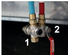
1. Drain plug for emptying the cold water circuit.
