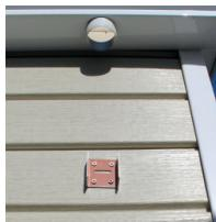
*Fit the gutter downpipe into its bracket.*
