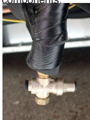
Connect the mains to the 15/21 male fitting located under the floor of the mobile home.
