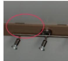
Air vent hidden under ceiling apex fixture
